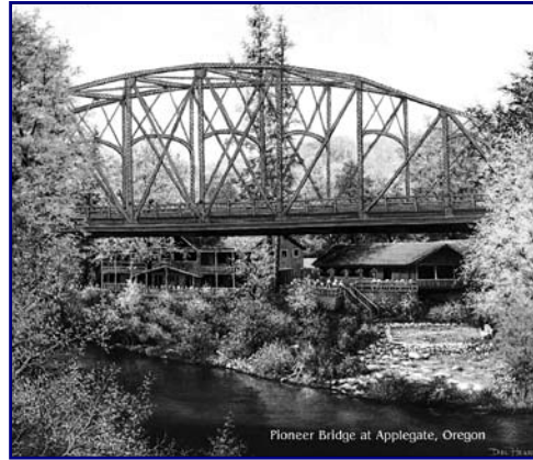
Pioneer Bridge at Applegate, Oregon
