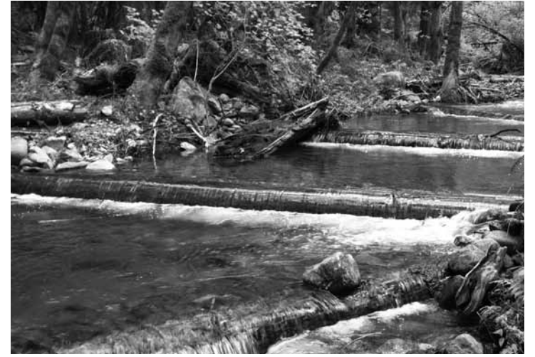
A large-wood installation on the west fork of Williams Creek. Photo by Chas Rogers.
