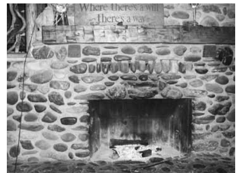
Stone fireplace in the lobby.
