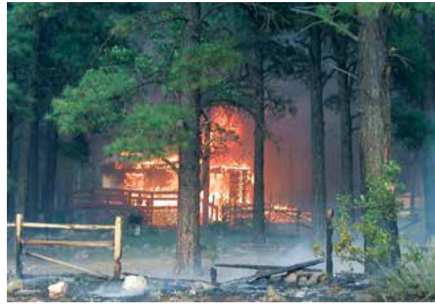
This home ignited due to fine fuels around it during the 2002 Missionary Ridge Fire in Colorado.
