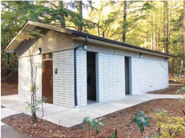
Newly restored restroom at Cantrall Buckley Park. Photo: Steve Lambert, Jackson County Parks.
