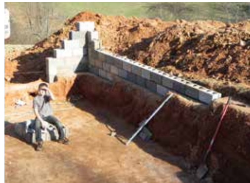
Photo, left: Consider native stone, cinder blocks or concrete for walipini walls (permies.com).
