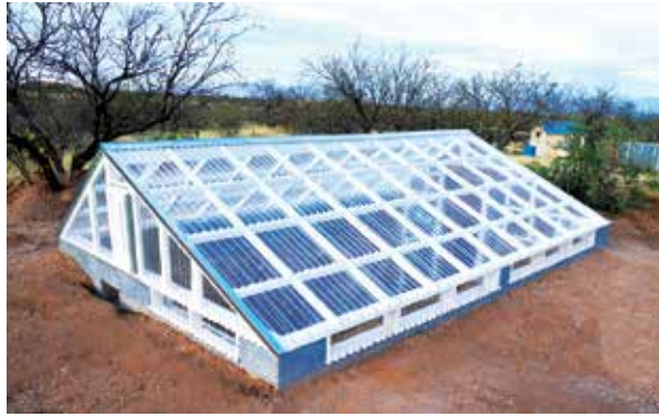
Cover your walipini with plastic or glass panels (i.ytimg.com).
