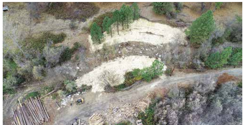
After: Forest Creek Project at the Ruch Sawmill, in October 2018.
