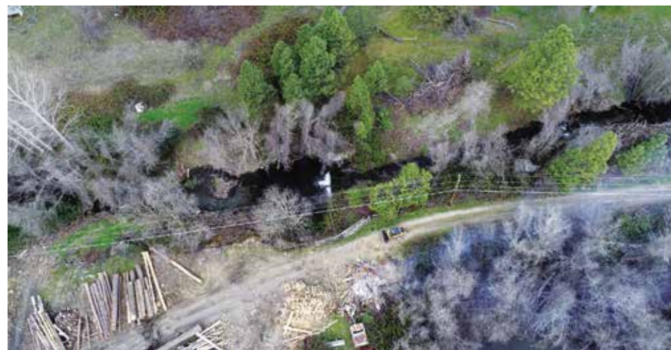
Before: Forest Creek Project at the Ruch Sawmill, in March 2018.
