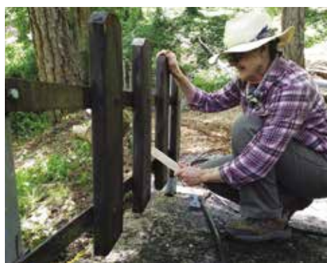
Hands-on chair, Janis Mohr-Tipton, scrapes footbridge pickets after power washing. Photo: Karin Barclay.
