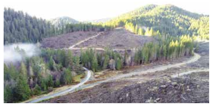
Logging operation on a tributary on the West Fork Evans Creek watershed.
