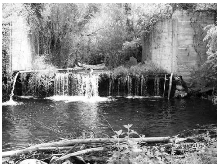
Before. Forest Creek dam obstructed fish passage—adult fish had to jump several feet; juveniles couldn't advance. Photo: ODFW 2005.
