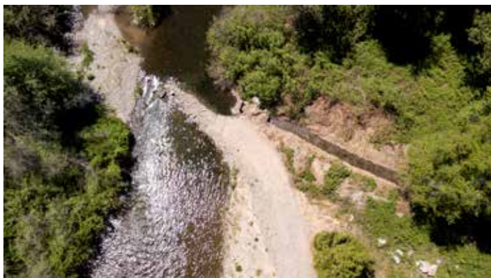
This view shows the push-up dam in place. Gravel would be piled into the creek each spring, raising the water level to reach the height of the irrigation ditch. Photo: APWC.
