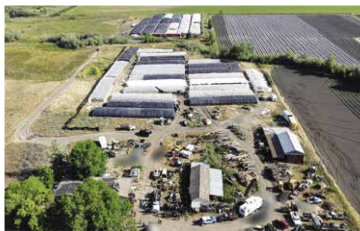
An aerial view of a black market hoop house near Central Point raided by a multi-agency task force in July. Similar operations in the Applegate are being targeted for code violations. Photo: Jackson County Sheriff’s Office.
