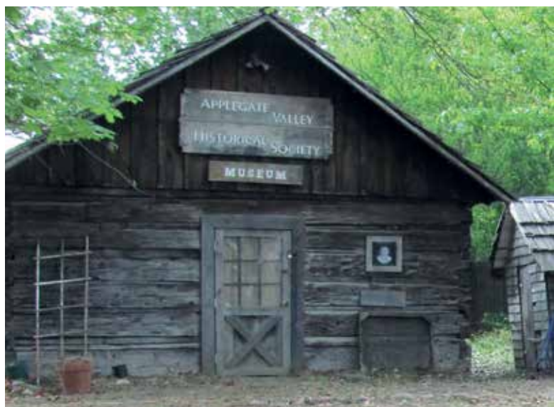
The old Applegate Store in the early 2000s after it was moved out of Jacksonville.
