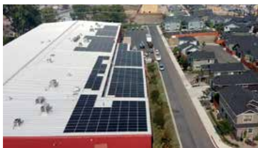
Energy from solar panels installed on the Oregon Shakespeare Festival workshop building in Talent is distributed to nearby neighbors as part of a community solar project.
