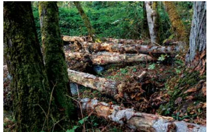
These Douglas fir logs were transported from the Provolt Recreation Site to Cheney Creek and “keyed” into trees on the stream bank to hold them in place.
