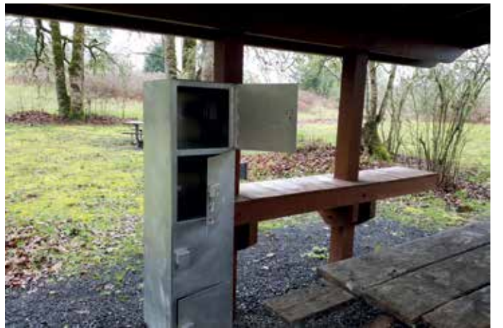
The new hiker-biker site for Cantrall Buckley Campground is modeled after this unit at Champoeg State Park in the Salem, Oregon, area. A partial wall will be added behind the counter for weather protection, as well as a pitched roof for better wind-resistance in our area. Photo: Janis Mohr-Tipton.
