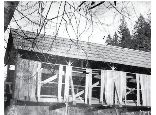
Huge trees carried by flood waters caused extensive damage in February 1927.
