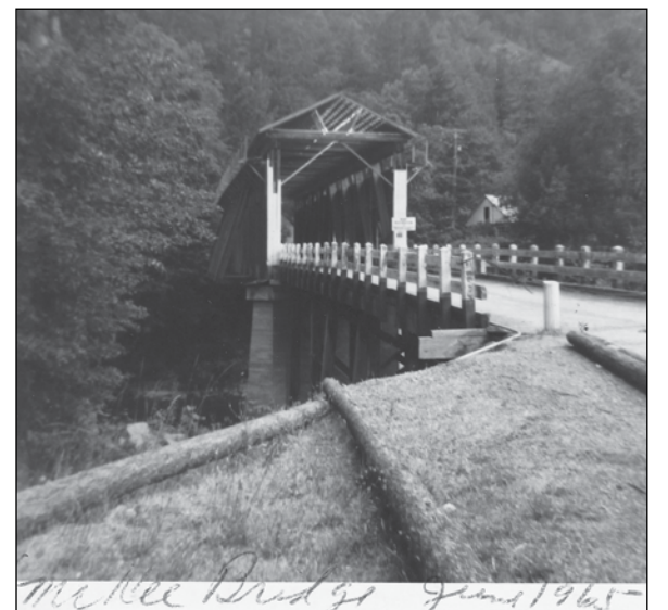
The roof was replaced after the Christmas Floods of 1964.
