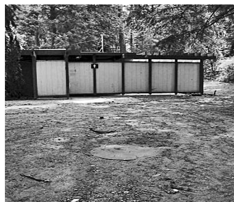
Photos: Top—Treatment wetland excavation with equalization tank in foreground and control building in background; Middle—New main power panel in campground; and Bottom—"D" area restroom showing pump access for new septic tanks.
