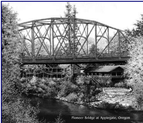
Pioneer Bridge at Applegate, Oregon
