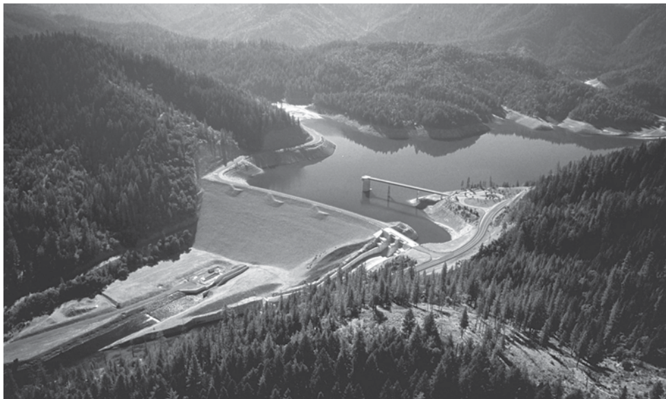
Applegate Dam looking south.
