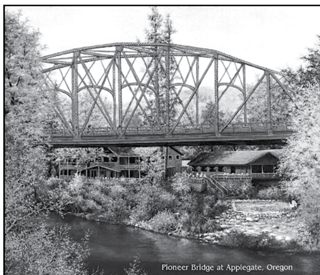
Pioneer Bridge at Applegate, Oregon
