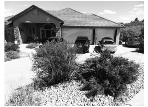
A nice, neat, safe, stucco house.
