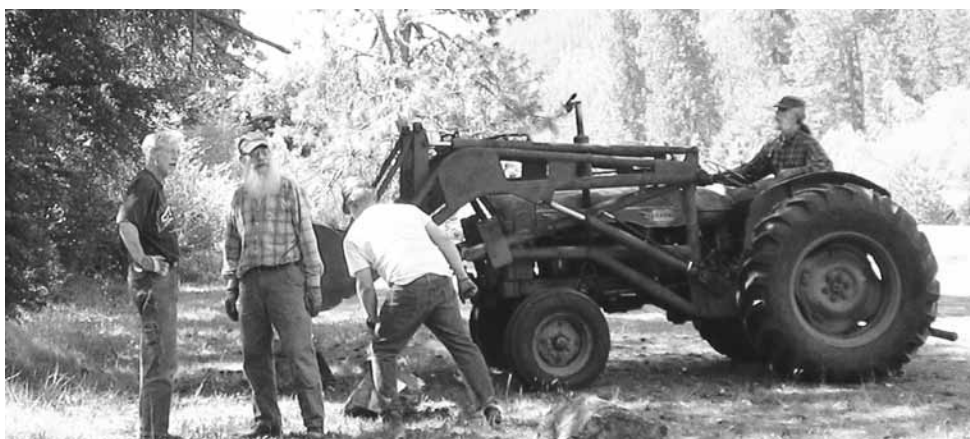
Jack Duggan, Paul Tipton, Peter Sturm and John Unger (on his tractor) created a rock barrier to protect the drain-field area in front of the Grange building.
