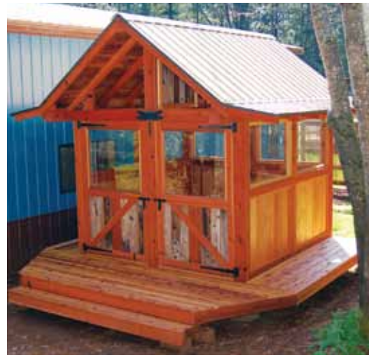
The Dragonfly Teahouse is made partially from reclaimed timber from the demolition of some Oregon mills.
