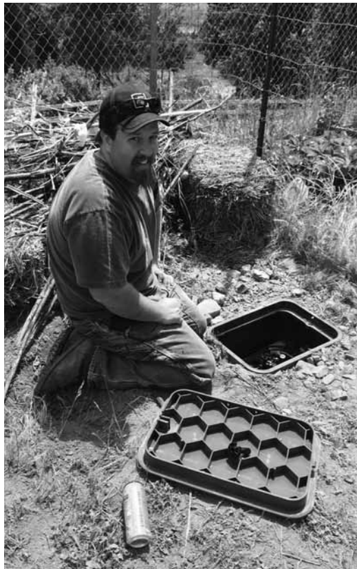
Photos (top) Joshua Morrison helped design and install the new irrigation system. (bottom) Tyler Van Buskirk used a trenching machine from his own business.
