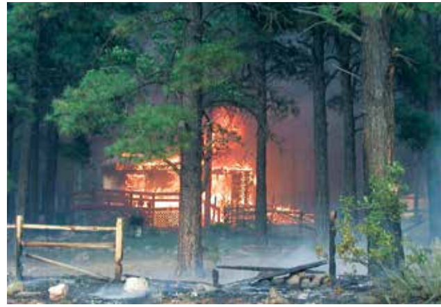
This home ignited due to fine fuels around it during the 2002 Missionary Ridge Fire in Colorado.
