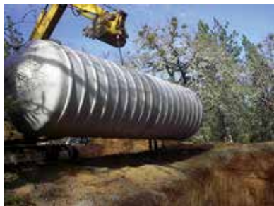
2007 installation of new septic tank.
