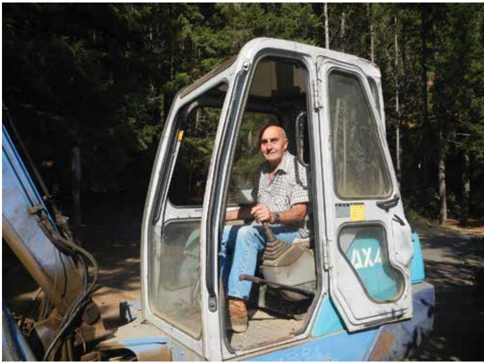
Tuffy Decker prepares the ground for the new playscape.
