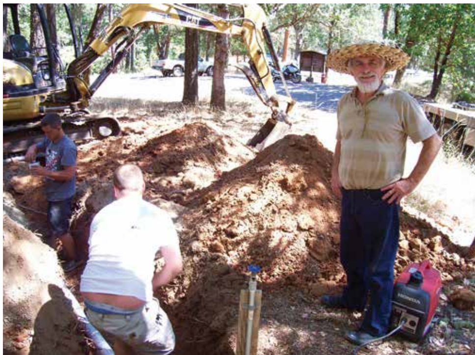
Laird Funk supervises installation of new electrical hookups in the campground.
