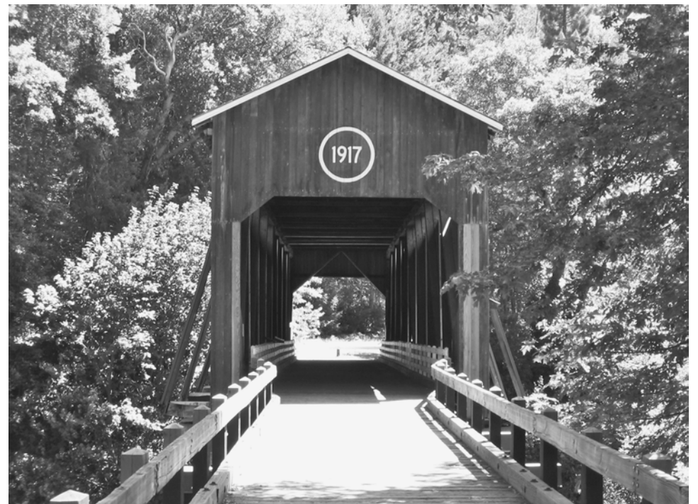
If you look closely at the white rails on the sides of the McKee Bridge, you might be able to see the camber (upward arch). Photo: Paul Tipton.
