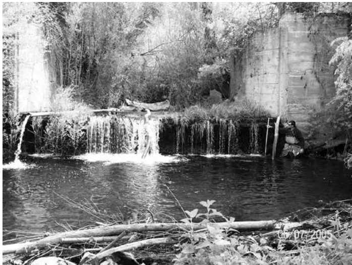
Before. Forest Creek dam obstructed fish passage—adult fish had to jump several feet; juveniles couldn't advance. Photo: ODFW 2005.
