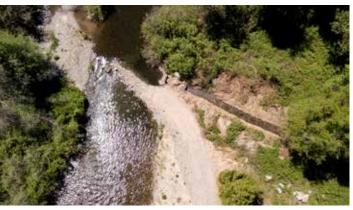
This view shows the push-up dam in place. Gravel would be piled into the creek each spring, raising the water level to reach the height of the irrigation ditch. Photo: APWC.
