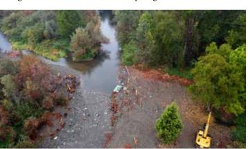
This shows the project site during construction. The dam has been  $exttt{dams}$  and  $exttt{other}$ removed and the irrigation headgate has been installed. The bare diversions on area on the right shows where gravel has been dug each year to build creeks and streams the pushup dam. This area will revegetate slowly over time. throughout the
