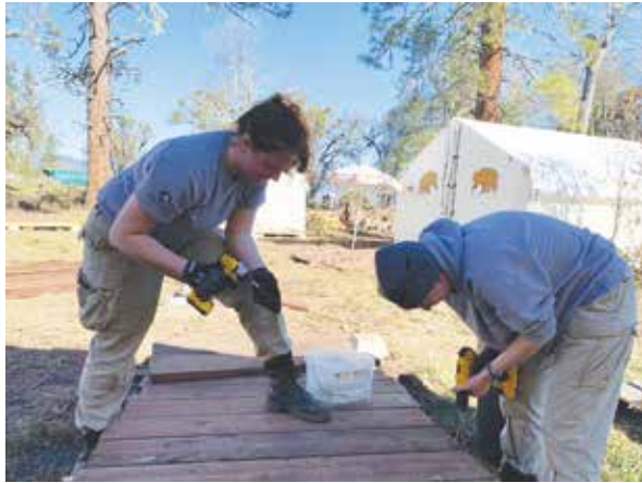
AmeriCorps crew members work on a boardwalk.
