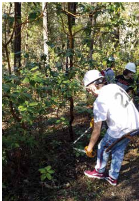
This student is determining the horizontal clearing line and removing limbs and small new growth that is in the tread zone. They also learned the vertical clearing limit for this trail in the campground.
