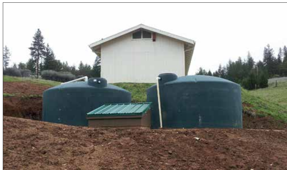
A 10,000-gallon rainwater collection system.
