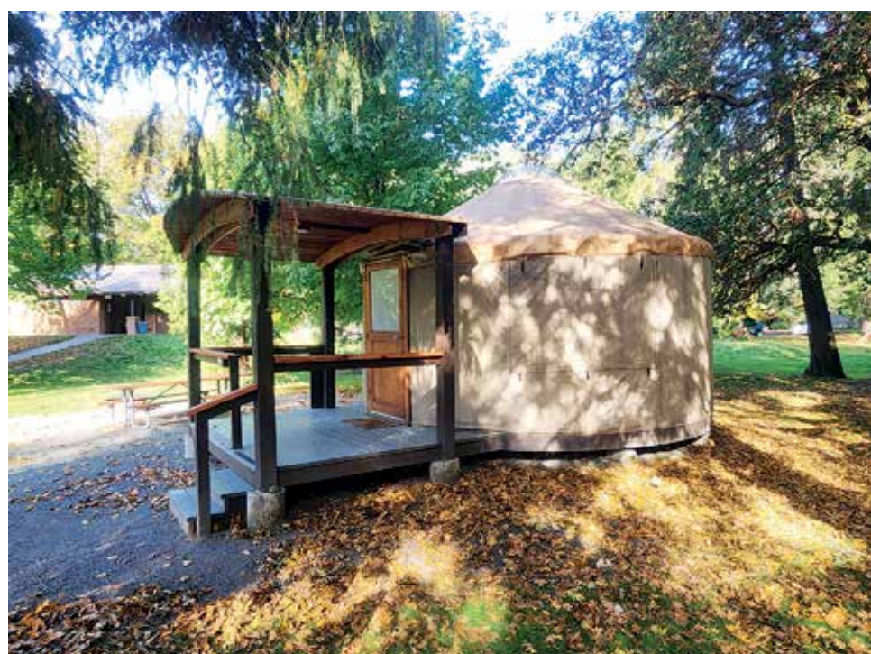
A new 16-foot Pacific Yurt installed at the Valley of the Rogue State Park. These yurts are available for the public to rent year-round on a reservation basis.
