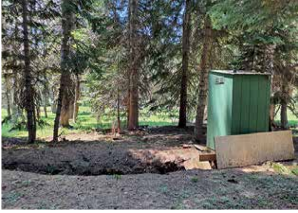
Illegal outhouse and trench built adjacent to Tamarack Meadow. Photo: US Forest Service.
