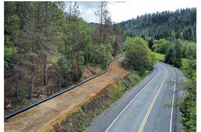
Irrigation pipeline ready to be buried along Little Applegate Road. Photo: APWC.
