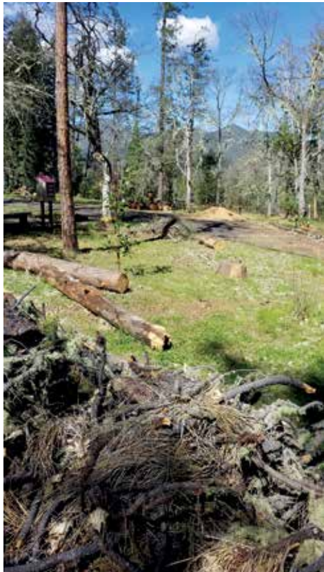
Dead hazard trees in Area B near the parking area were removed for safety. Photo: Janis Mohr-Tipton.
