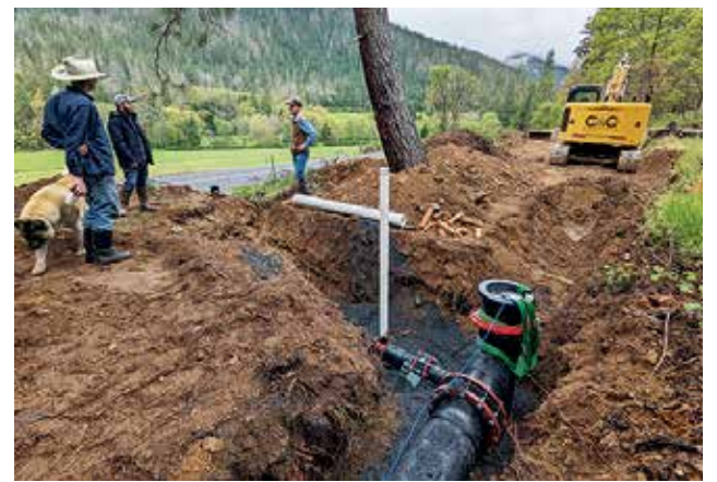
JSWCD engineer Paul DeMaggio explains the new turnouts to irrigators. Photo: APWC.
