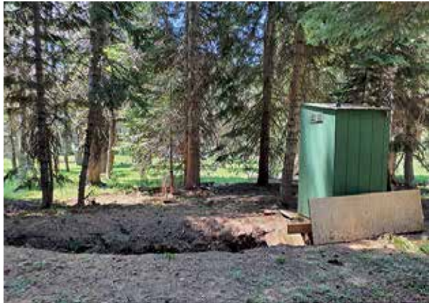
Illegal outhouse and trench built adjacent to Tamarack Meadow. Photo: US Forest Service.
