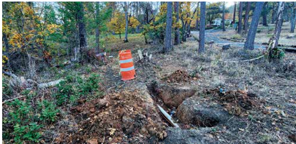
Park personnel are in the process of opening up valve intersections and replacing electric valves with air-pressure valves. Photo: Janelle Dunlevy.
