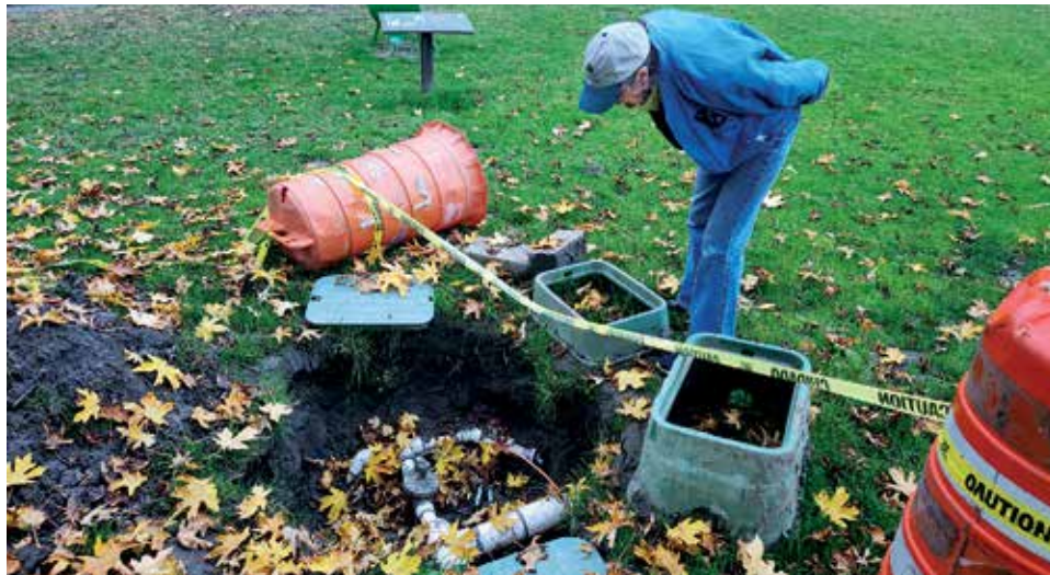
Janis Mohr-Tipton, APWC volunteer park enhancement committee chair, examines the work needed to replace the large valves for the eight-inch pipelines required for irrigation. Photo: Janelle Dunlevy.
