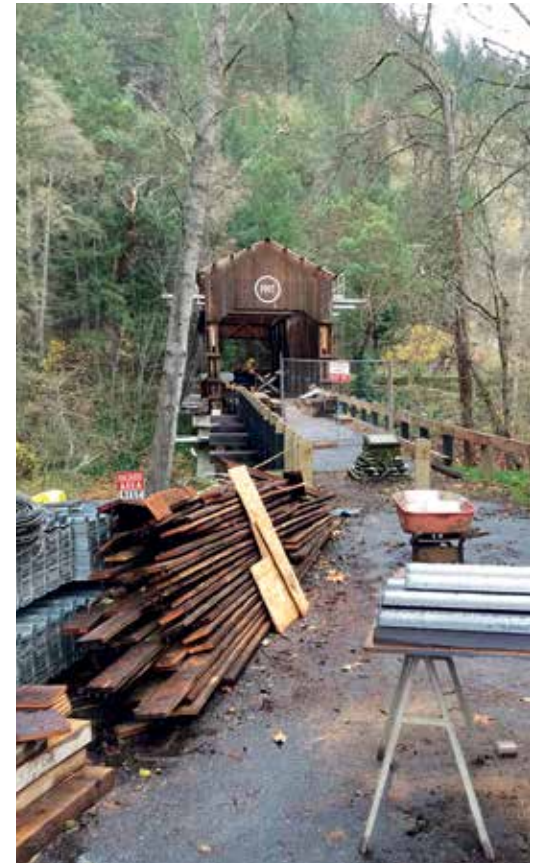
McKee Bridge under renovation.
