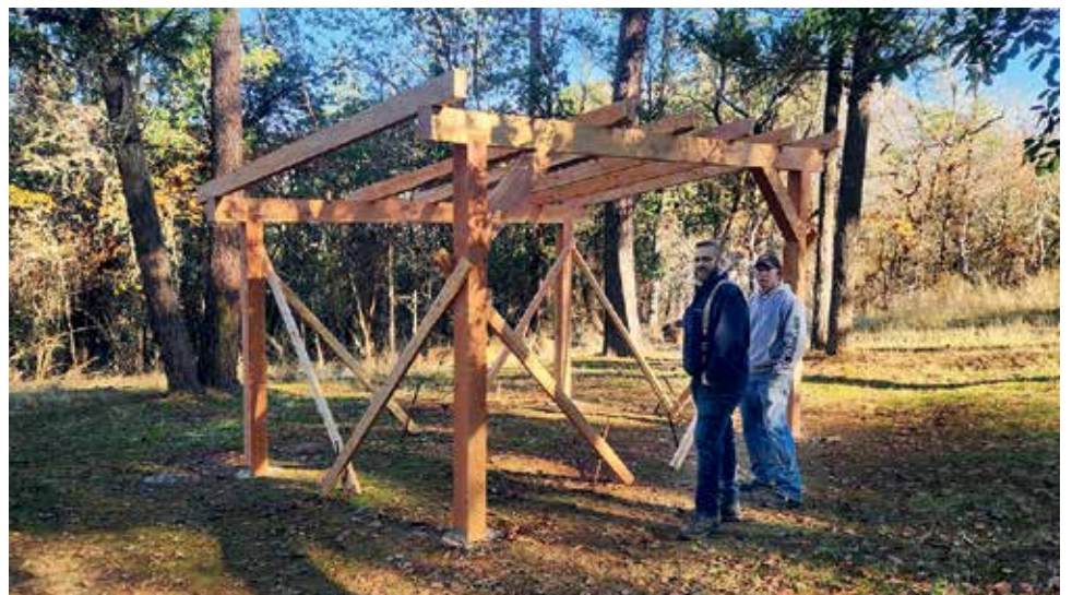
Tom Maddox (left) and Cody Goodnough working on the Hiker-Biker Shelter, which was constructed by local contractors using dead trees harvested from Cantrall Buckley and milled locally by 4M Timber. Photo: APWC.
