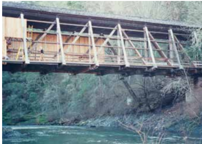
New siding on McKee Bridge in 1995.
