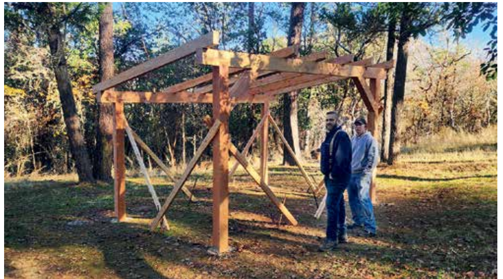
Tom Maddox (left) and Cody Goodnough working on the Hiker-Biker Shelter, which was constructed by local contractors using dead trees harvested from Cantrall Buckley and milled locally by 4M Timber. Photo: APWC.
