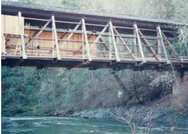
New siding on McKee Bridge in 1995.
