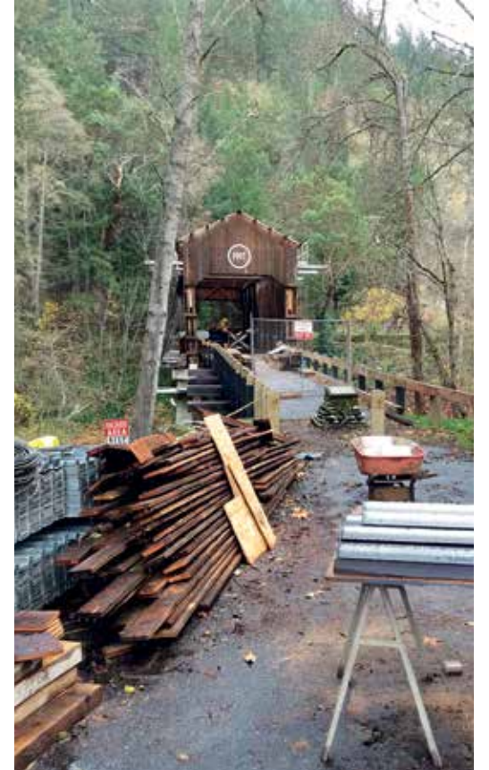
McKee Bridge under renovation.
